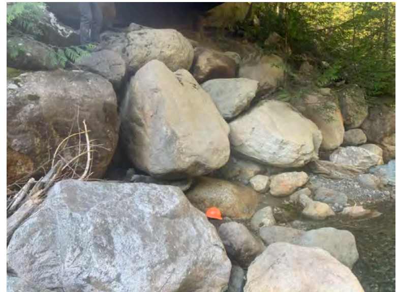
Left Bank Abutment when facing downstream
