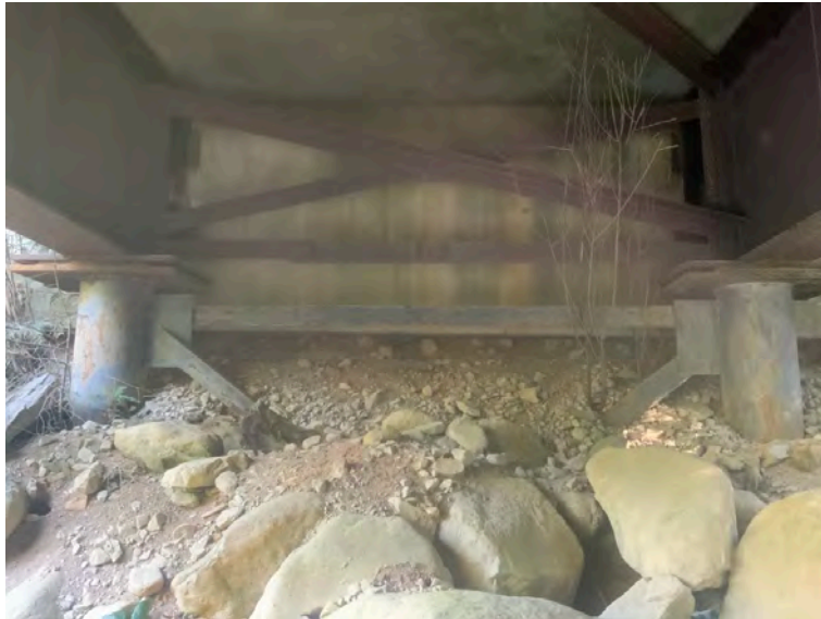
Right Bank Abutment when facing downstream
