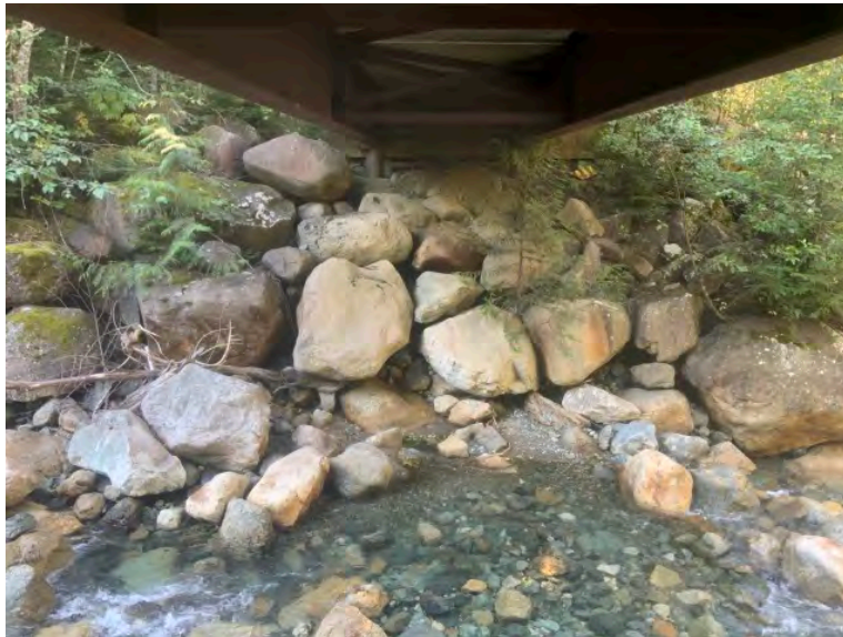
Left Bank Abutment when facing downstream
