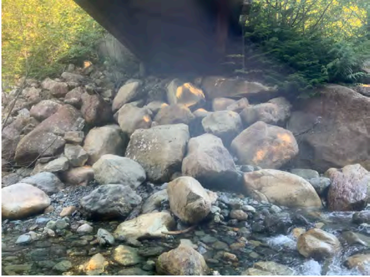
Right Bank Abutment when facing downstream
